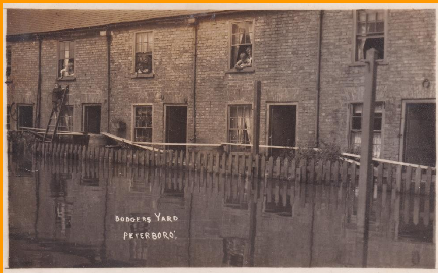
Floodwater in Bodgers Yard, Peterborough
